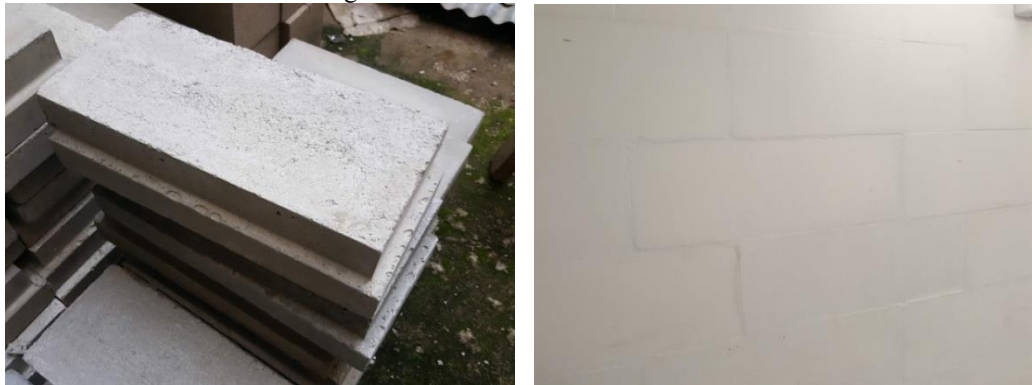
FIG. 15. Concrete blocks for 'sacrificial' layer
