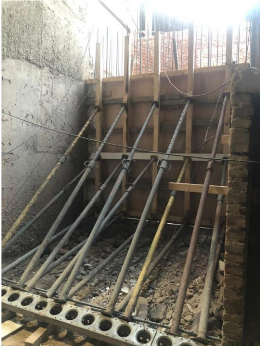
FIG. 10. Shoring system to extern vault wall
