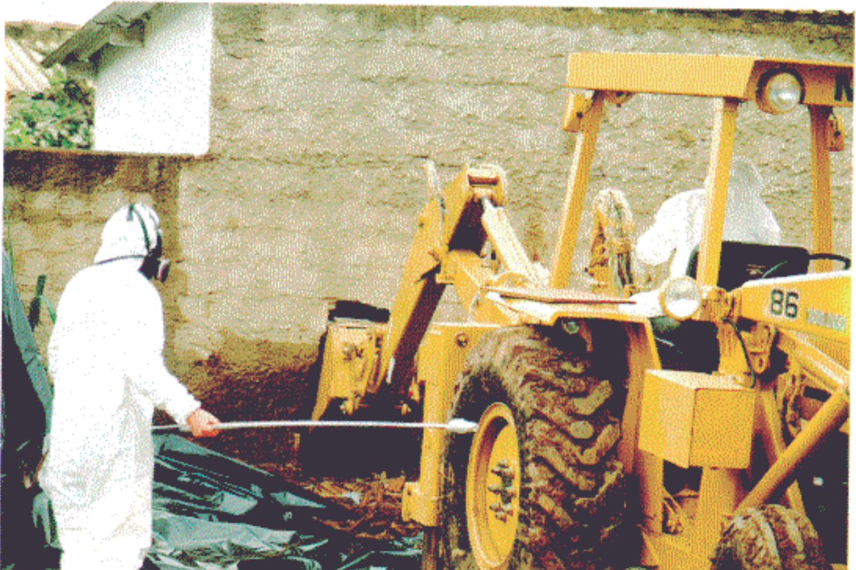
Demolishing work: dose rates up to 0.5 Sv/h
