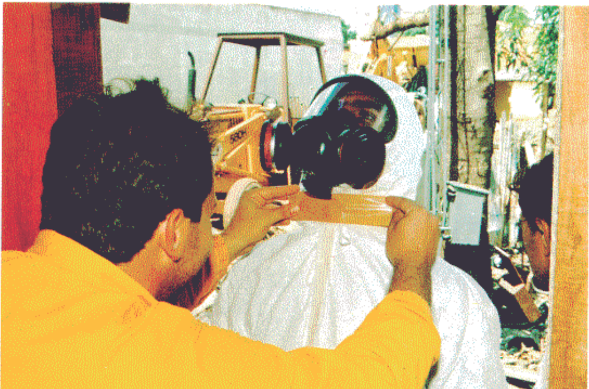
Preparing to demolish the contaminated houses
