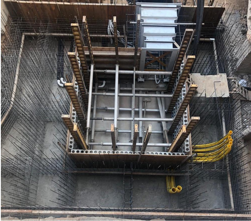
FIG. 6. Wooden frame inside the armor previous the concrete cast
