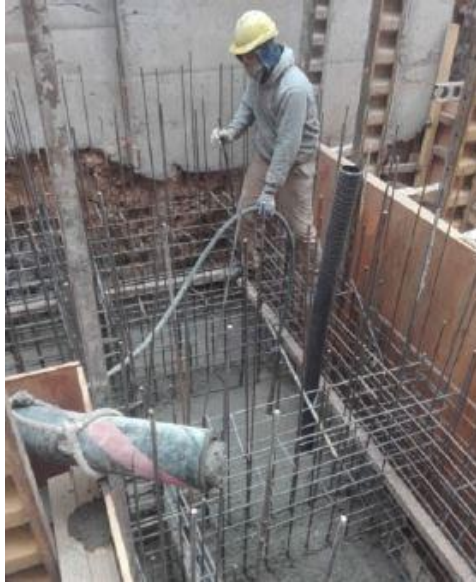
FIG. 9. A civil worker vibrating the concrete during the cast
