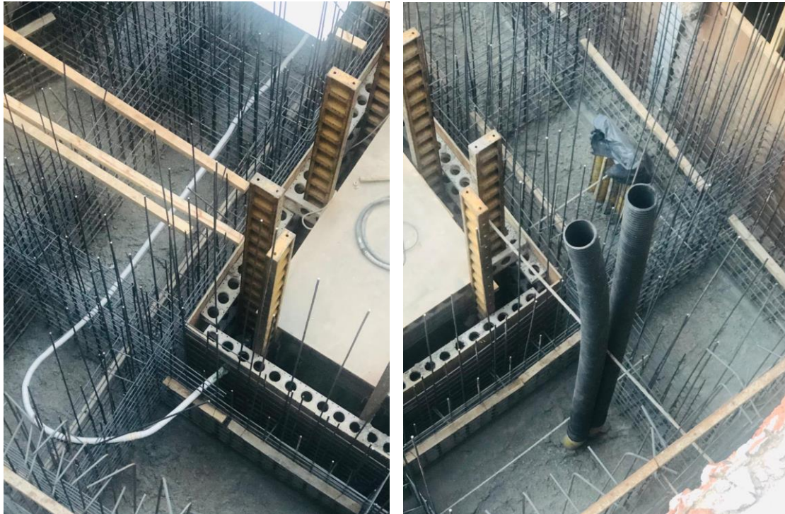
FIG. 12. Absence of intern metallic tensors
