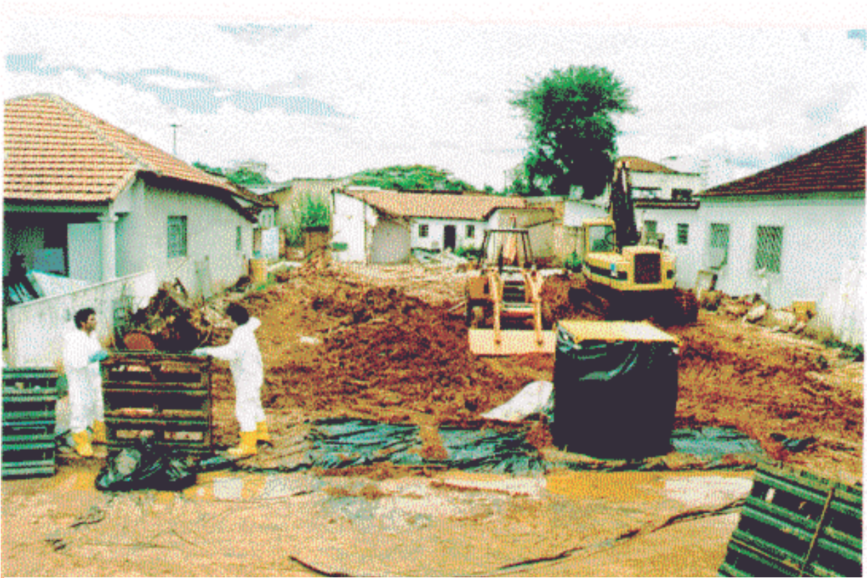
Restoration after removing the contaminated rubble
