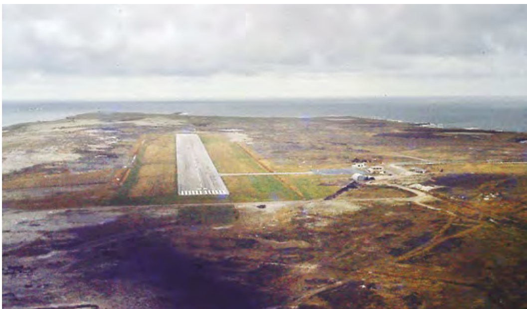
Stanley airport runway finished - Photo courtesy of: Com. (R) Canosa
