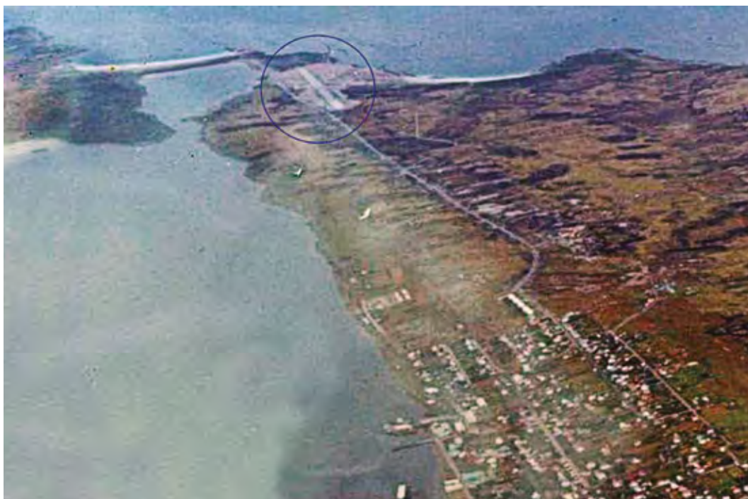
The aluminium airstrip, build by Grupo 1 de Construcciones at Hookers Point, 2 km Stanley Port
