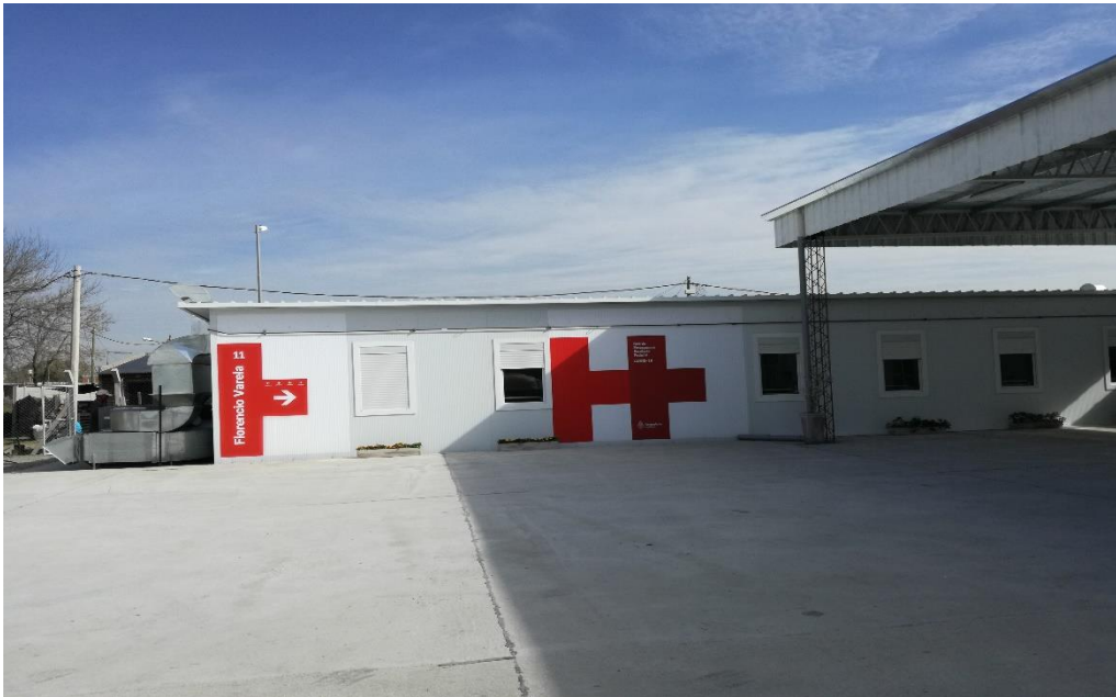
Hospital modular, PBA
